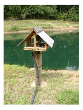
This custom-made HUT to the left is positioned well above the dam's highest point so it is not possible for high water to damage the compressor unit. The hut's roof guards well against any heavy rain while allowing any heat generated by the electric motor to blow away in the breeze.
